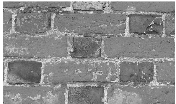
Brick pattern called Flemish Bond using burnt headers
